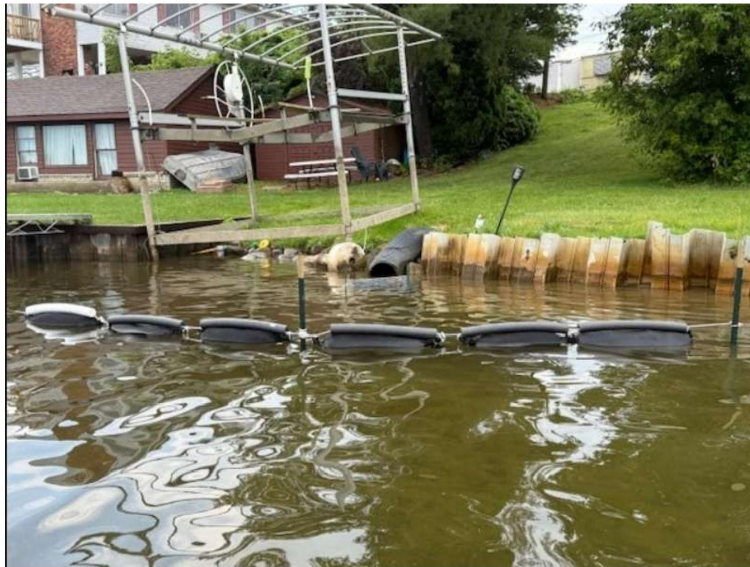
Picture 1 of 3 showing Timber Char around 15 inch drain from Meier's parking lot directly into the lake.
